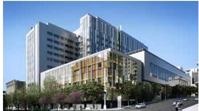
Geary Van Ness Medical Center in California was the first structure in North America to use Viscous Wall Dampers.
